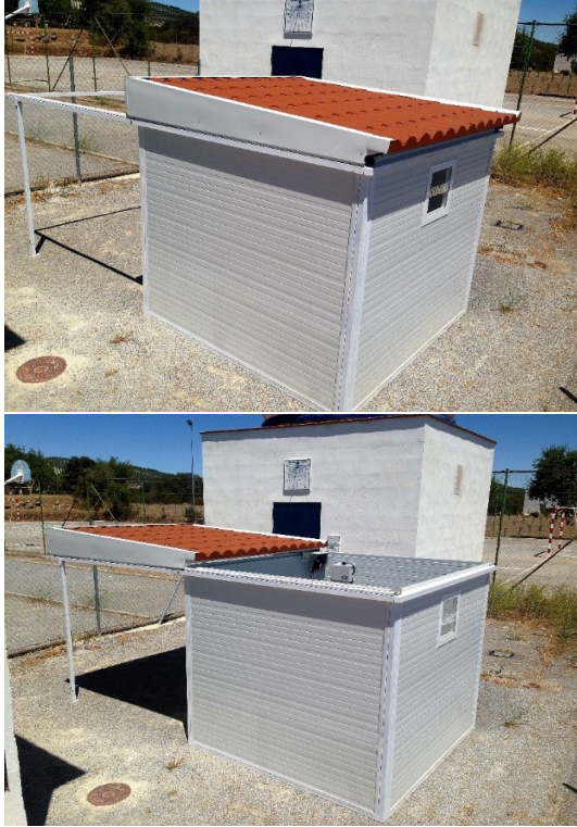
Fig. 1. PROAM Observatory in open/closed positions
