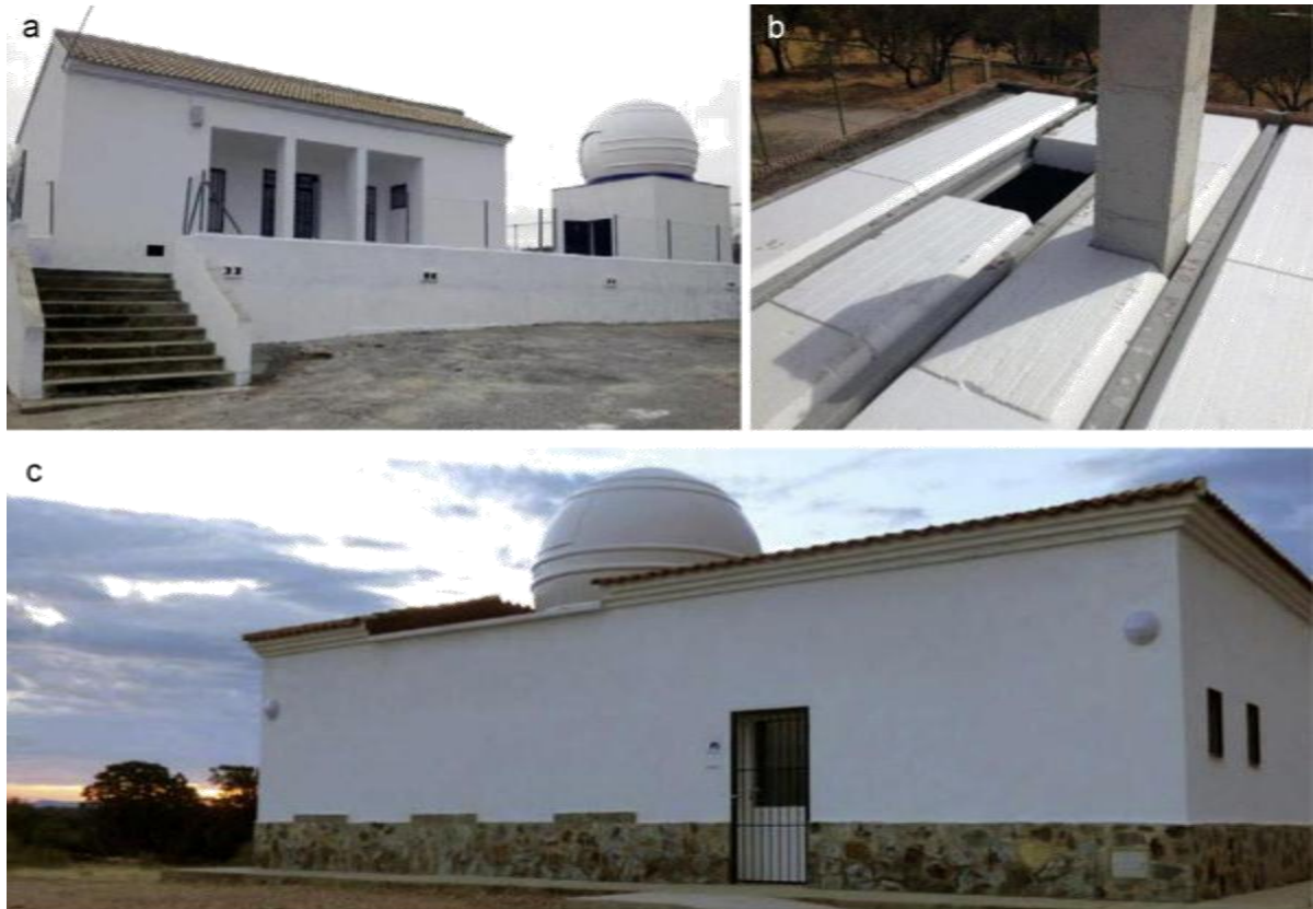
Figure 3. a) Observatorio Andaluz de Astronomía finished, b) Detail of the floor and pillar of the telescope, c) Observatorio Astronómico de Mongragüe finished.
