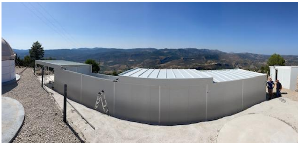
Figure 2. Image of AstroCamp hosting with an open roll-off roof (right). The roof on the left is closed.
