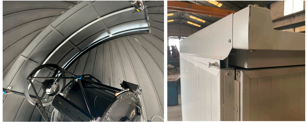
Figure 6. (Left): Interior detail of RSO showing the satin black fireproof primer. (Right): Detail of the cover/running rail design with external overlap that allows air circulation and prevents water and snow from entering (ProAm Robotic Observatory).
