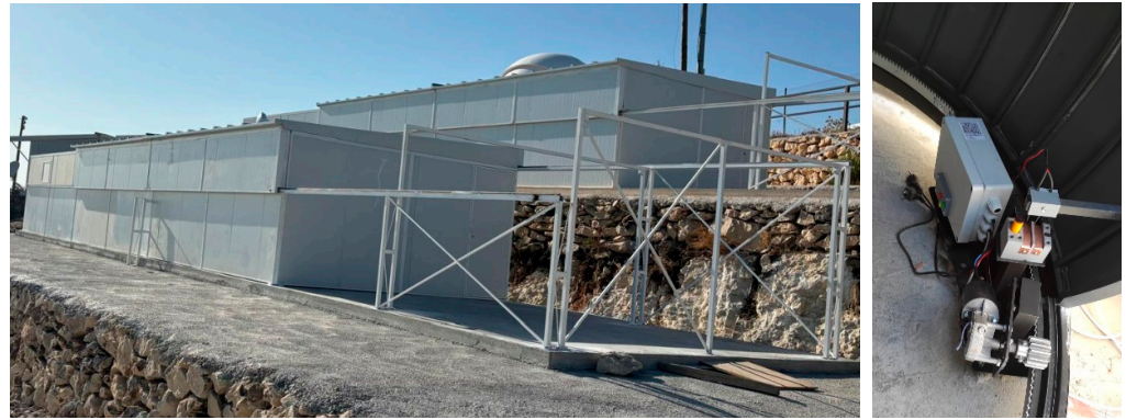
Figure 5. (Left): Roof and walls made of laminated steel sandwich panels with polyurethane interior at the AstroCamp Observatory https://www.astrocamp.es/ (accessed on 14 December 2025). in Nerpio (Spain). (Right): Rack-and-pinion motor system with variable speed drive and manual/remote control electronics box.
